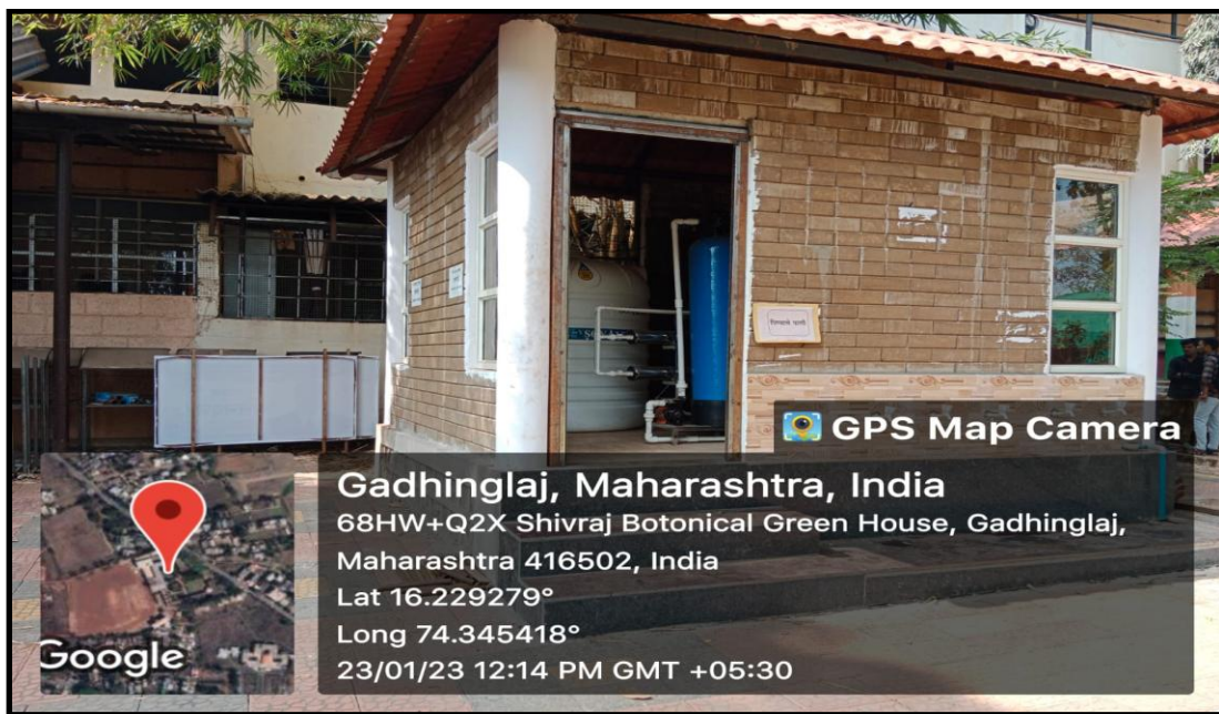
Purified Drinking Water Facility
