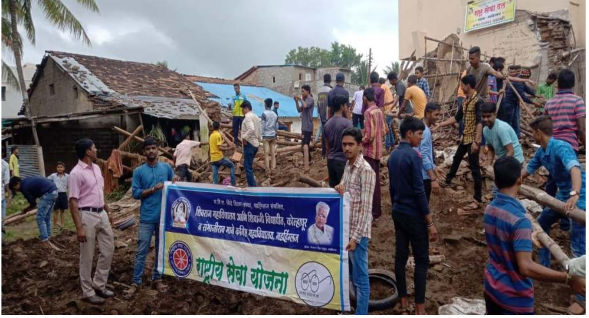
Cleaning Flood affected village Dundge
