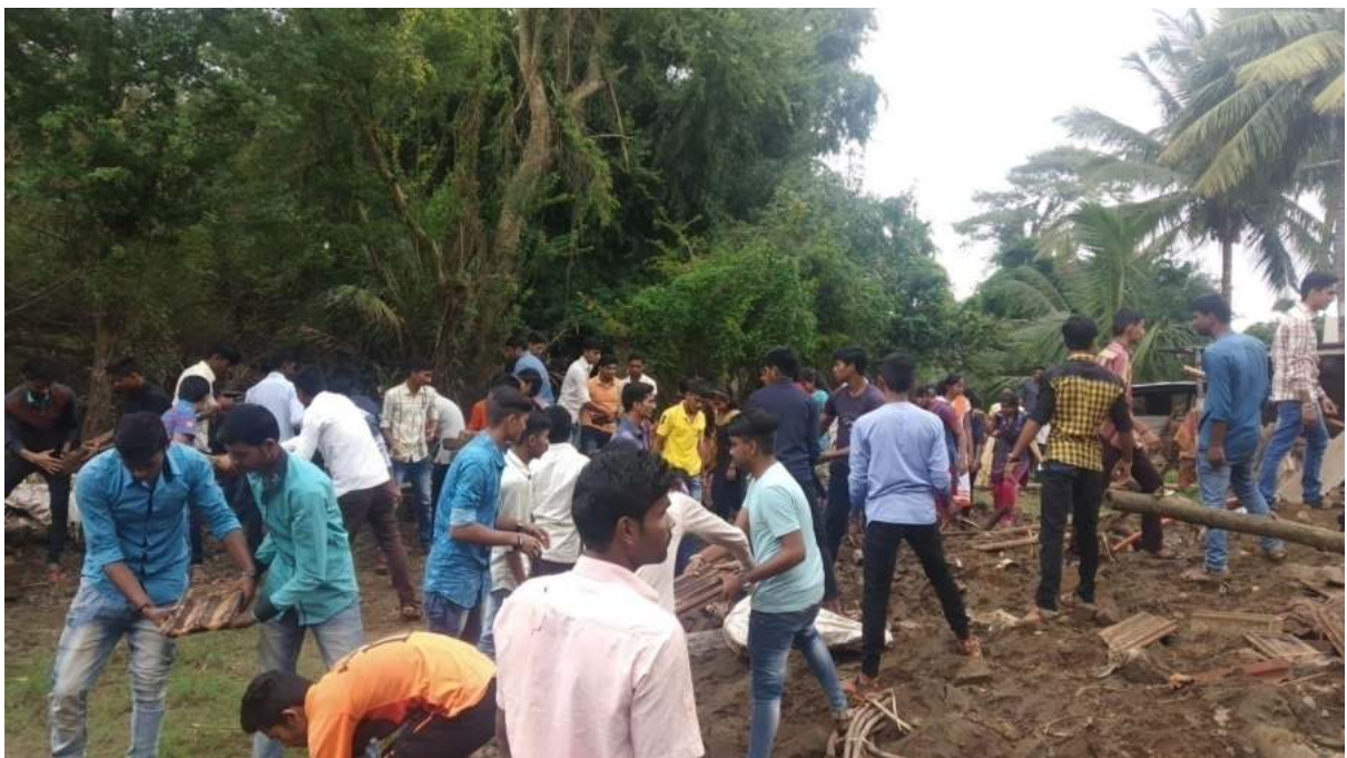
Cleaning Flood affected village Dundge
